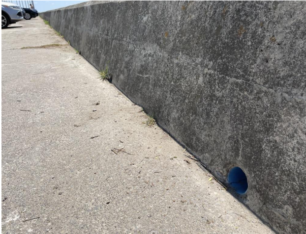
Figure 5 & 6. The stormwater runoff pipes are situated through the cement breakwall between the parking lot and swimming area that leads directly into Olympic Harbour Beach.
